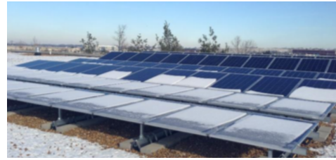
Figure 2: Flatter surface leads to more snow accumulation and longer snow melt time.
