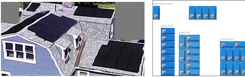
Fig. 1. A residential solar array (right) with 31 panels deployed on four roof planes and real-time panel-level generation data from the array (left).
